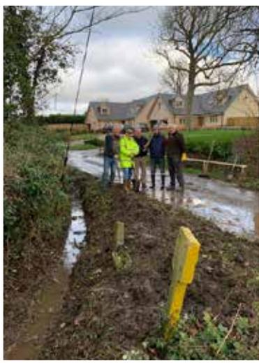
Our January working party met in Phoebe Lane to solve a problem. The new houses storm water together with the drainage from the recreation ground was causing a problem in the lane with large deep puddles and running water damaging the unmade road surface. The ditches and gullies were completely blocked and needed a
